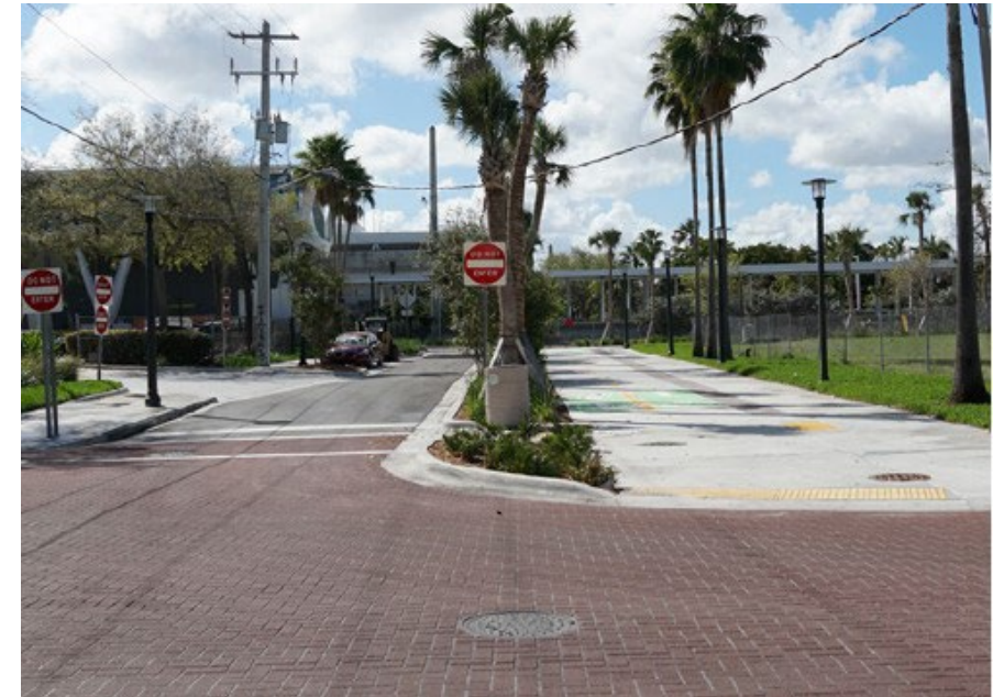
Downtown Fort Lauderdale Mobility Hub Streetscape improvements, including a two-way cycle track, pedestrian lighting, and ADA improvements. Source: Broward MPO.
