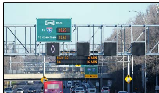
The image highlights the price to utilize the MnPASS lanes, which adjusts based on congestion, thus providing drivers with information with which to make travel decisions. Image courtesy of MnDOT.
