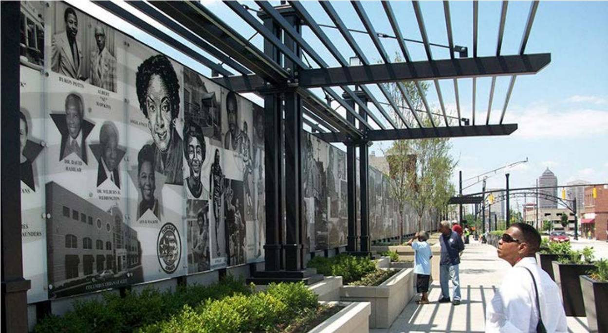
Cultural Wall on Long Street Bridge in Columbus, OH (Courtesy of ODOT)
