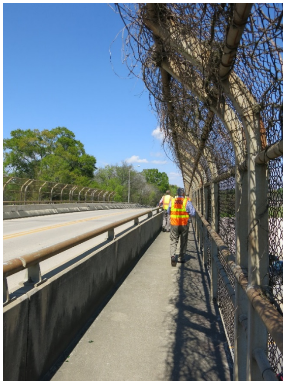
Sidewalk along East Side of Nairn Bridge (Photo Courtesy of Louisiana DOTD)
