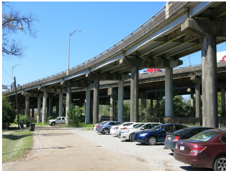
Parking adjacent to Perkins Road Ramps (Photo Courtesy of Louisiana DOTD)
