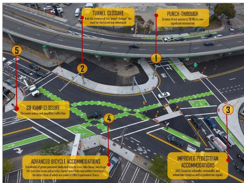
Improvements at the McCarthy Overpass and the intersection of Somerville Avenue and Medford Street (Courtesy of MassDOT).
