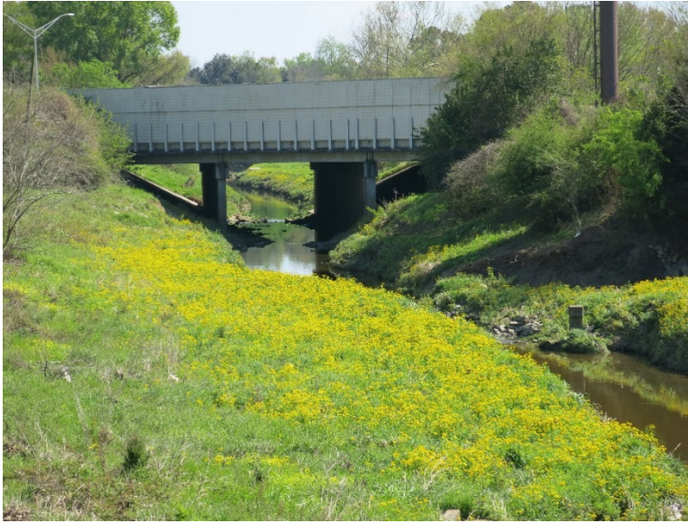
Ward Creek under I-10 (Photo Courtesy of Louisiana DOTD)
